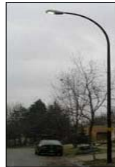
Photo of cobra head street light
