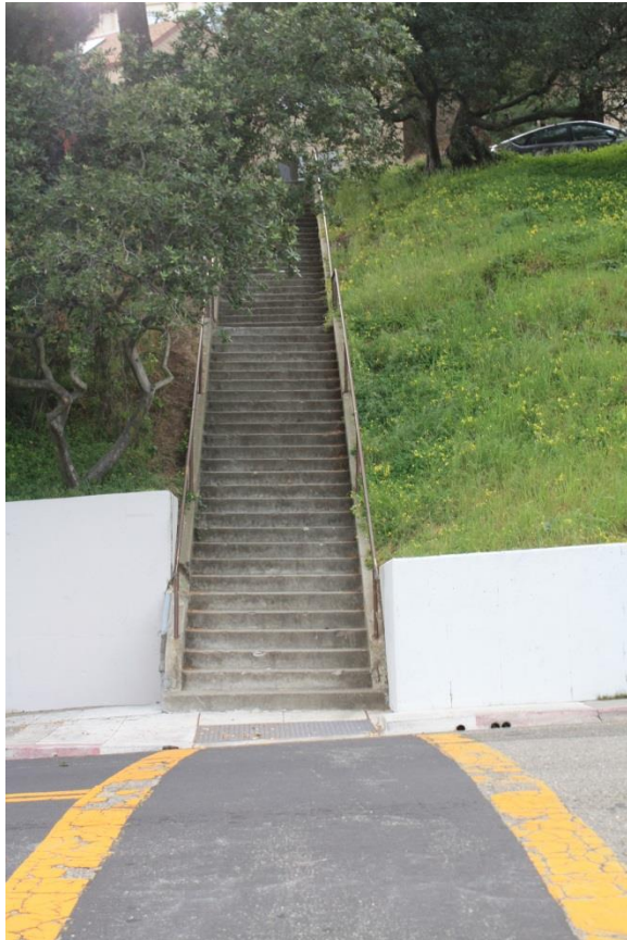
Stairway and crosswalk at Jackson Street near Castro Street
